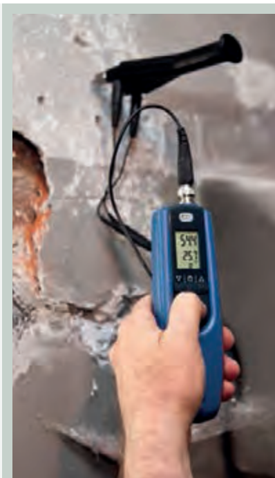
APPLICATION Measurement of plaster moisture using an M 20 electrode
